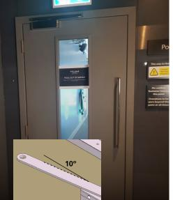
To overcome the issue preventing the doors being held completely shut, Rutland designers quickly created a modified version of the TS.11204 closer, changing the angle of its closer arm in the 'door closed' position. By increasing the angle from five to ten degrees, sufficient force was applied to ensure that the hotel's doors were held closed – notwithstanding the deeper architraves – and therefore fire safety compliant.
